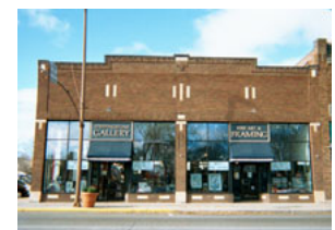
An example of a storefront revitalization from a grant program offered through the EDA in Hutchinson, one of the steps already taken by the city to reinvest in downtown.
