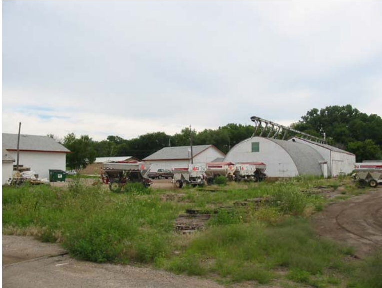
Site looking northeast from the Luce Line Trail
